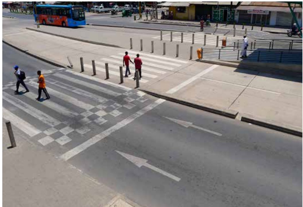
Figure 35. A tabletop crossing provides safe access to a BRT station.
