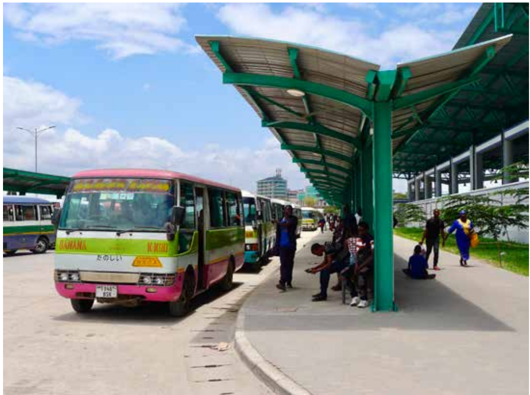
Figure 49. High-quality bus terminals offer protection from sun and rain, seating, and universal access.
