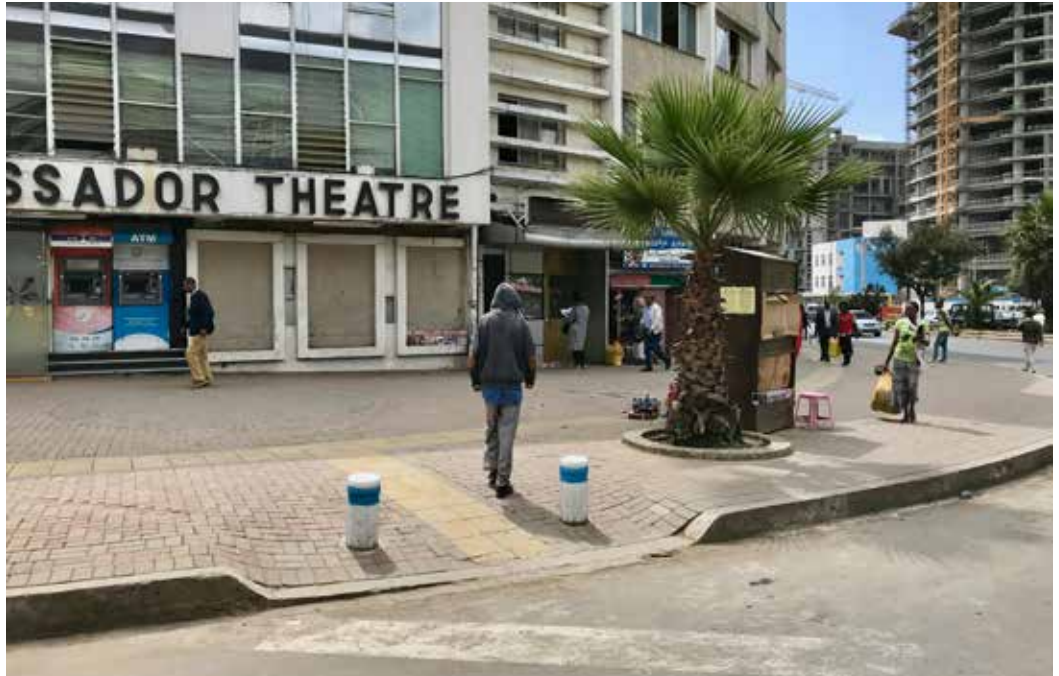
Figure 29. Footpaths should ramp down to the level of the carriageway, with a maximum ramp slope of 1:12.
