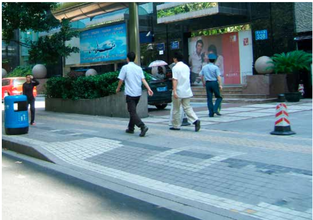
Figure 31. Property entrance treatment maintaining the footpath clear width at the same level.
