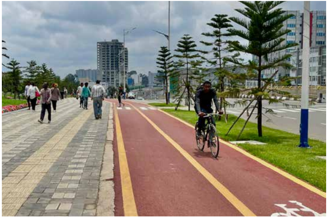
Figure 38. Newly constructed cycle tracks should be physically separated from motor vehicle traffic and raised +150 mm above the carriageway.
