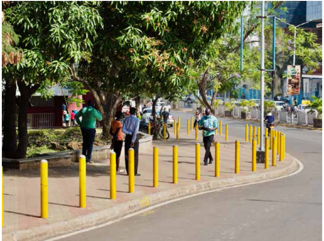
Figure 28. Footpaths placed below the carriageway often experience water-logging. Footpaths should be raised +150 mm above the carriageway.
